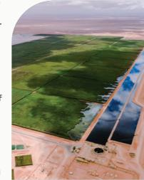
**BAUER Nimr water treatment** project is based on a nature-based solution that is inherently carbon neutral. It can effectively convert hydrocarbon contaminated water into clean recyclable water, plant biomass and a nutrient-rich organic soil improver, all without consuming any electricity or chemicals, while supporting the establishment of new habitat, enhancing biodiversity and climate resilience.
